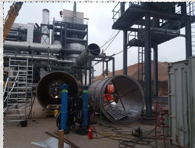
Assembly of flue gas ducts and compensators.
